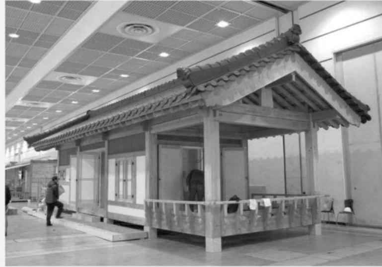
The prefabricated modular Hanok at the 2012 Seoul International Construction Fair
