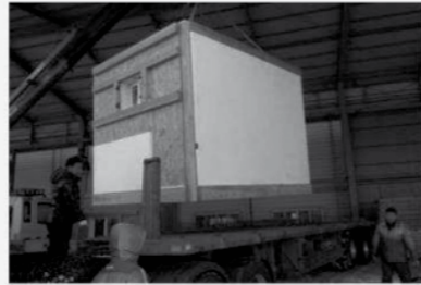
Assembly of the prefabricated modular Hanok
