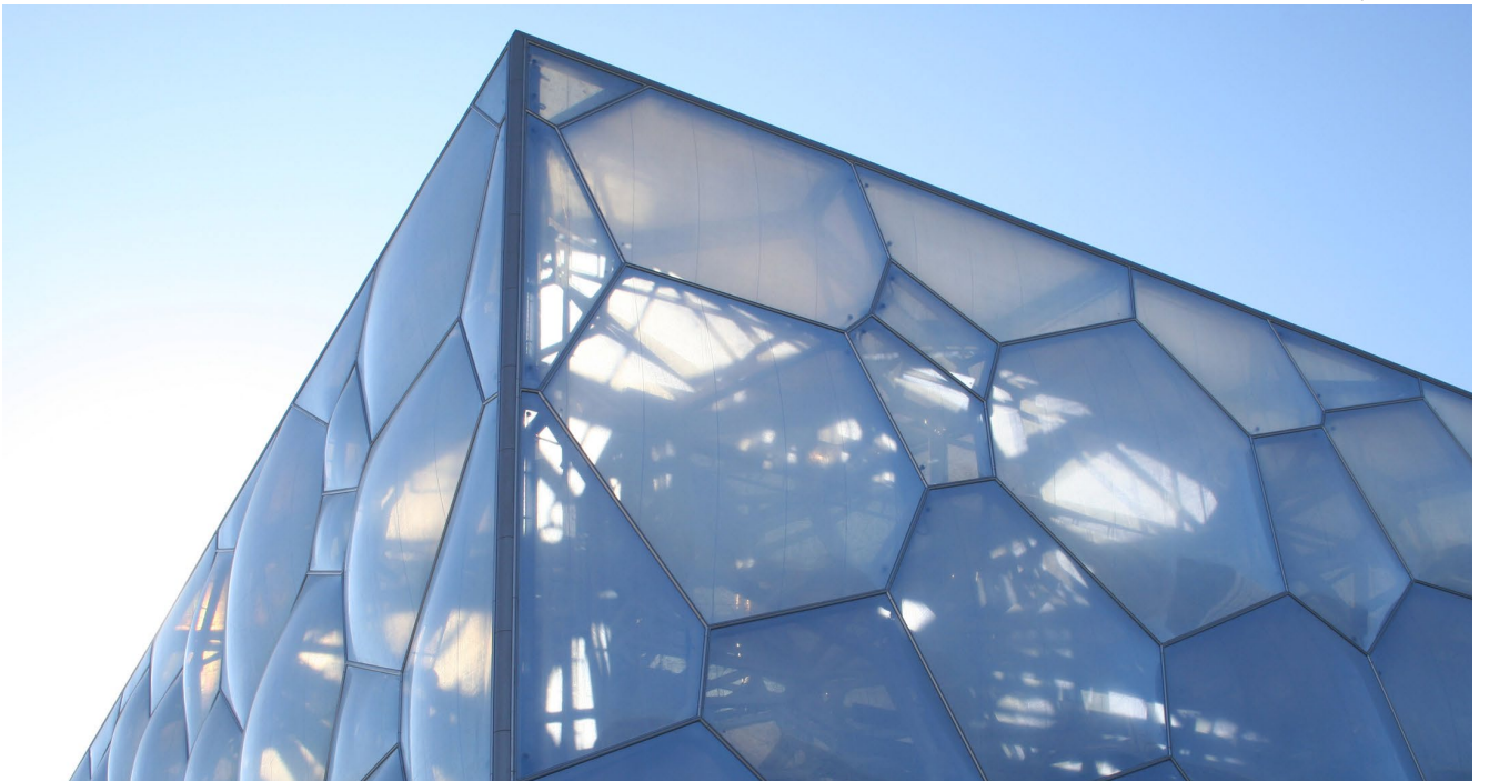
Abb. 59: Water Cube, Peijing
