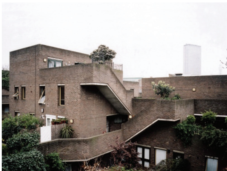
Abb.54: Odham's Walk, Innenansicht [50]
