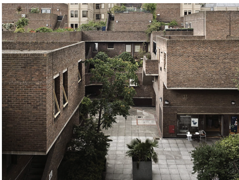
Abb.53: Odham's Walk, Innenansicht [51]
