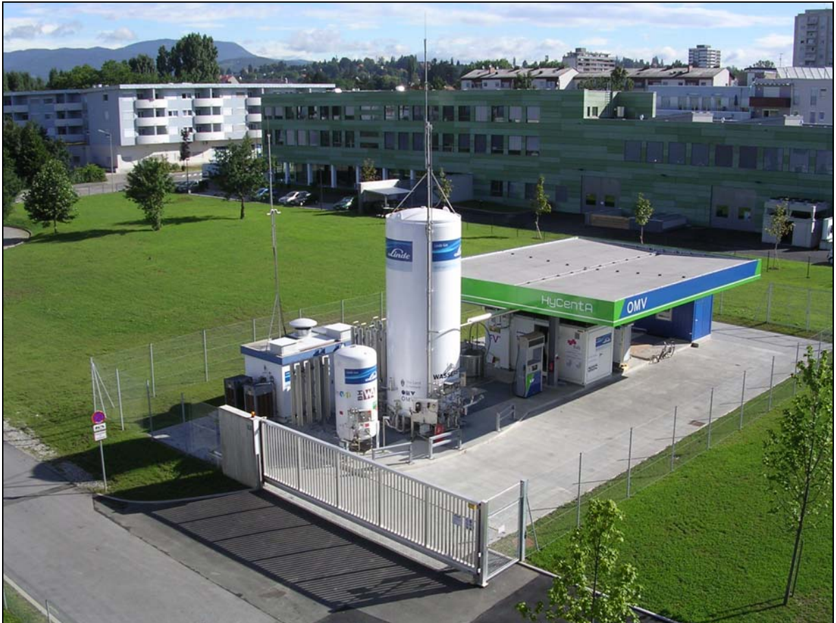
Figure 32: Hydrogen refueling station TU-Graz 40
