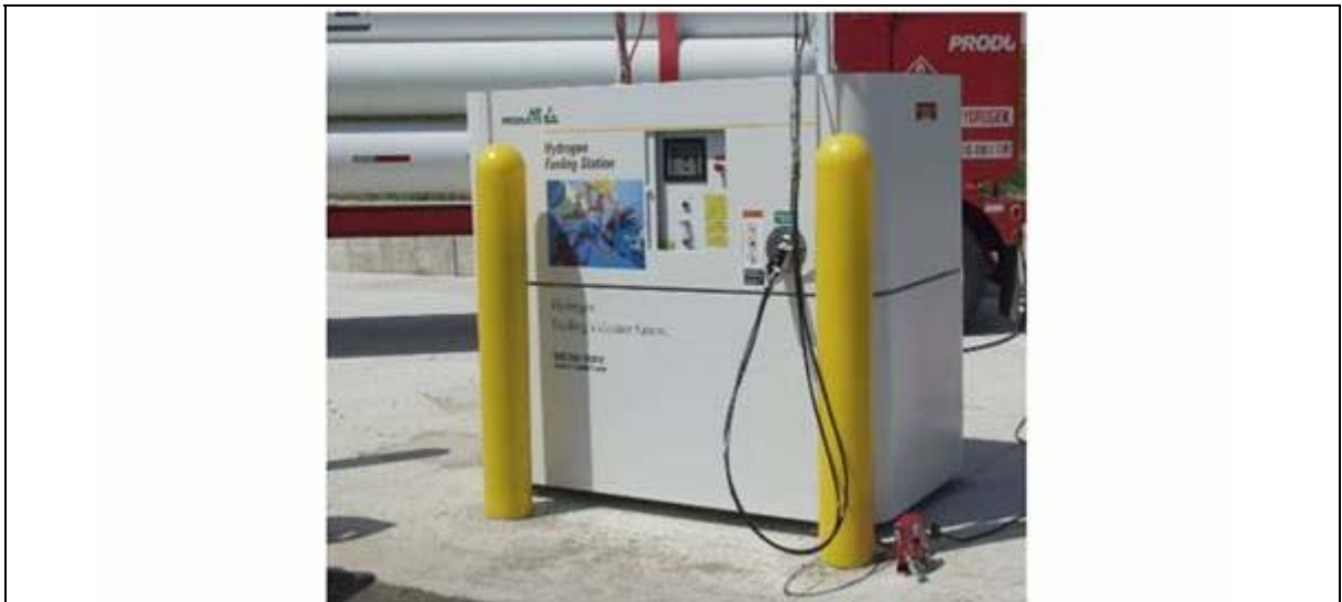
Figure 33: Air Products Series 100 station 42
