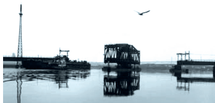
Image Source: The Pennsylvania, New Jersey and New York Railroad Co. Portal Bridge along the Northeast Corridor Railroad line in an undated photo, looking south towards the Pulaski Skyway. The swing bridge is open to permit the passage of a barge. Extracted from the NJMC Masterplan 2005 edited by Andreas Huemer
