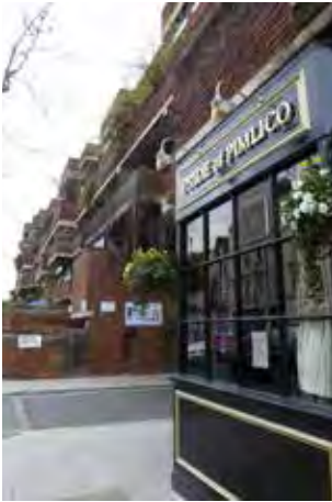
fig 214: Playful facade and one of the three public houses
