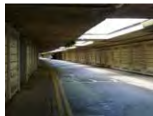
fig 201: Below ground car park
