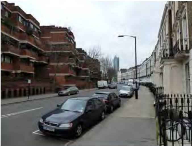
fig 215: Lillington Gardens is based on typical proportions found in the surrounding fig 216: impressions of the circulation areas
