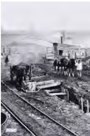
fig 43: Constructing the below-grade portions of the Embankment
