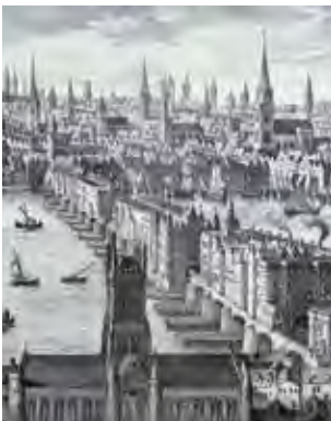
fig 18: London Bridge from 1209. Some of the houses had up to seven stories and cantilevered off the bridge's edge.
