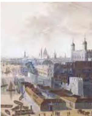
fig 26: A 1804 painting by William Daniell of the Tower of London with the busy Pool in front of it
