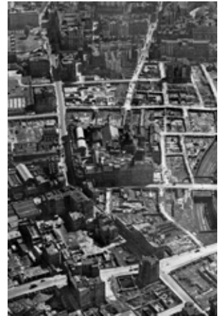
fig 153: War destruction on the future construction site
