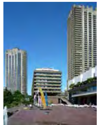
fig 154: Barbican Centre Terrace
