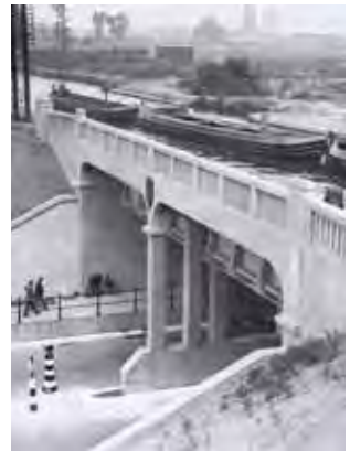
fig 45: In 1939, the Grand Junction Canal crossing over the new North Circular Road via an aqueduct
