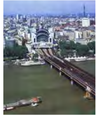
fig 54: The tracks into Charing Cross station go over the river. An office building was built above the station.
