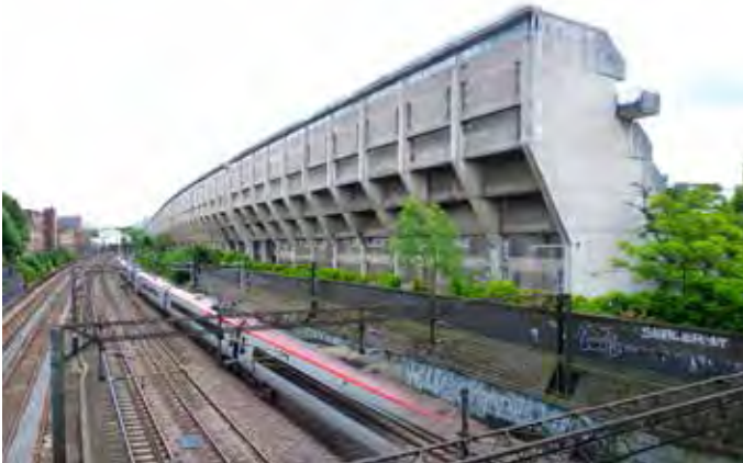
fig 189: The machine-like back of block A as a noise barrier
