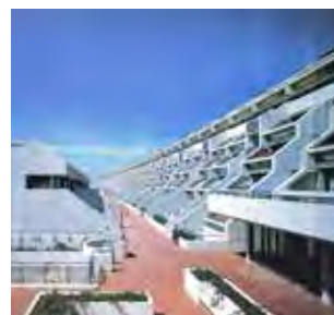
fig 204: Rowley Way at completion
