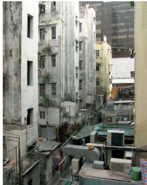
Abb. 5.21 Photo #9: Service Lane
