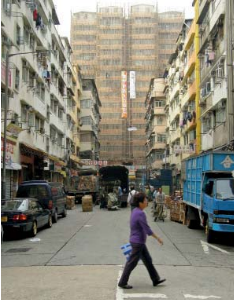
Abb. 5.18 Photo #6: Chun Tin Street
