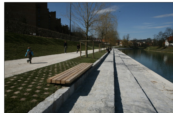
Illustration nr. 62 / The Trnovo Embankment after renovation
