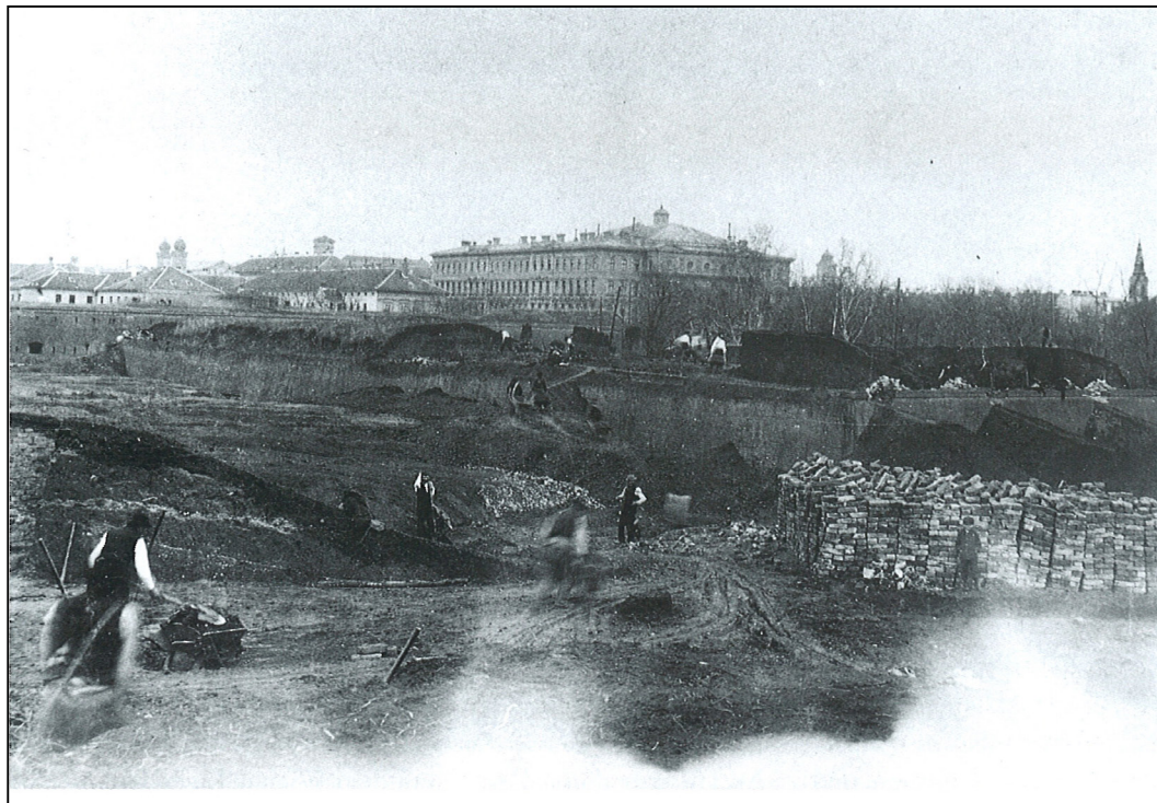
Illustration nr.20 / Timisoara – Demolition of the Fortifications
