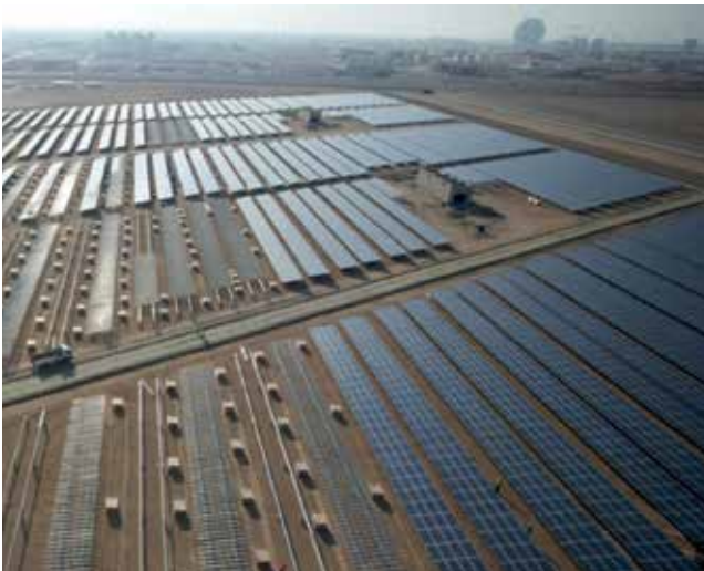
Abb. 4.6 Photovoltaikanlage Masdar City
