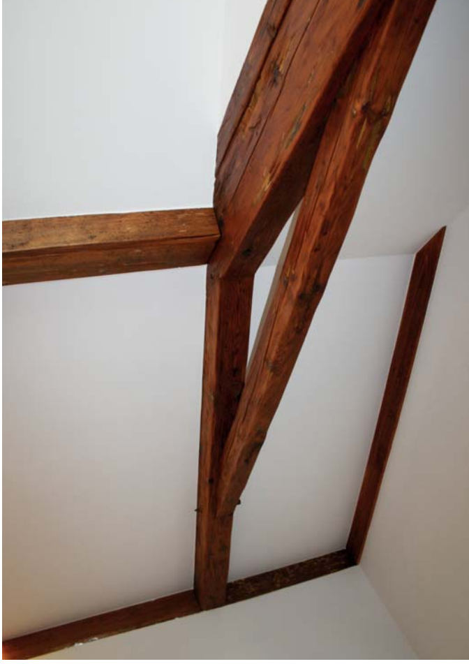
Abb. 163 links: Umlaufendes Gebälk / surrounding mature timber
