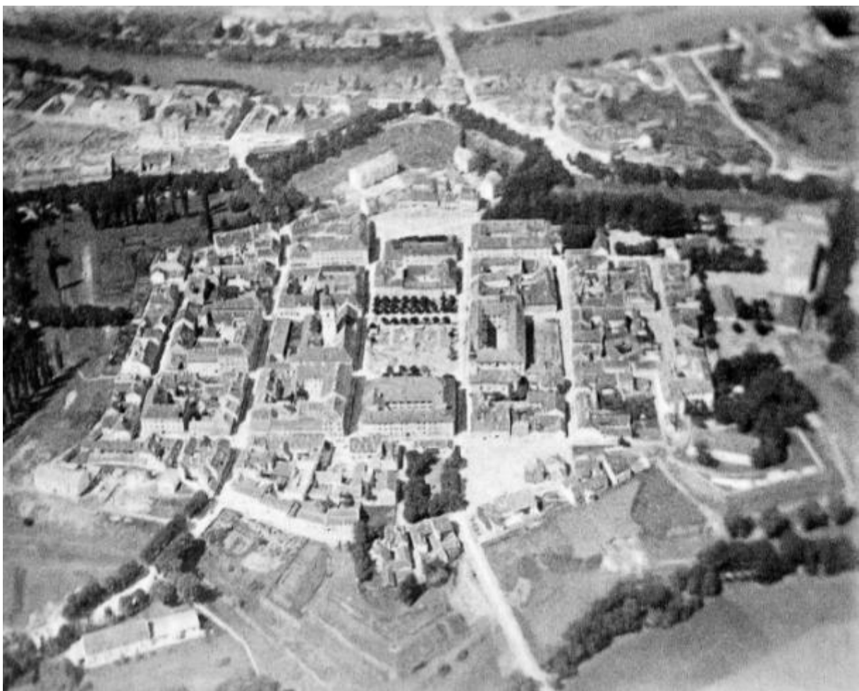
Figure 34, Aerial view of the Karlovac “Star”,KA-Fotka, 1930
