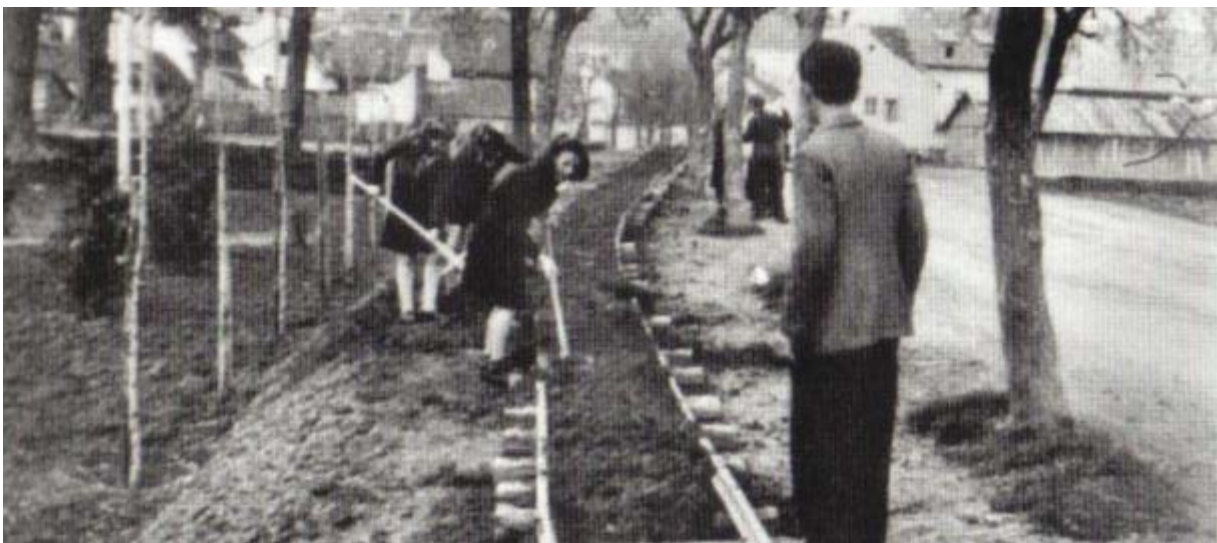
Figure 38, The reconstruction of the “Ruski Put” Street, KA-Fotka, 1951
