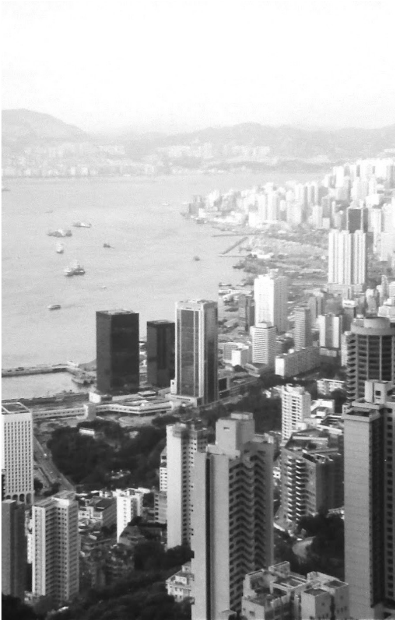
fig.12 View to North Point, 1984
