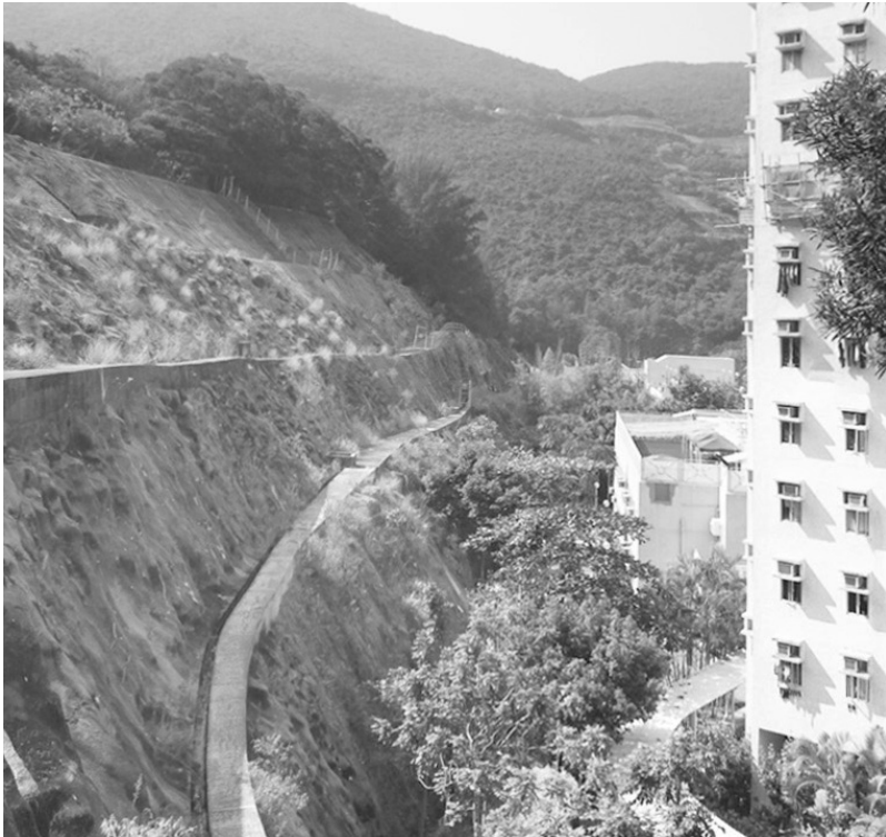
fig.58b typical cut-slope formation next to estate
