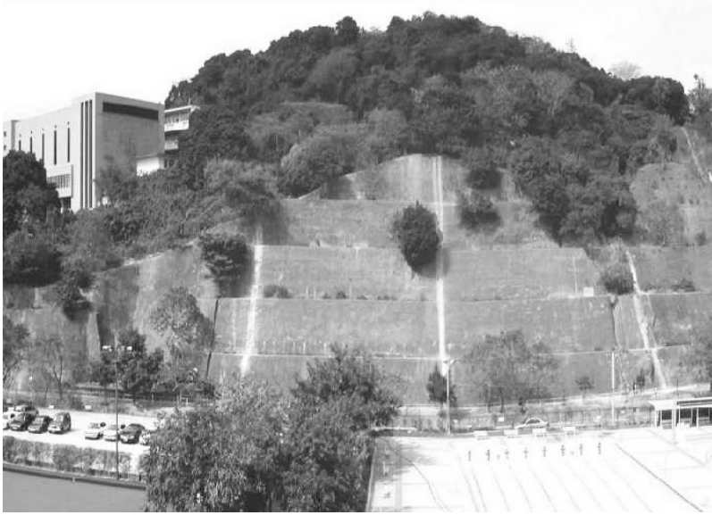
fig.58a typical cut-slope formation next to infrastructure
