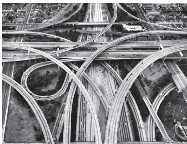
A.K.A. 'Spaghetti Junction'
