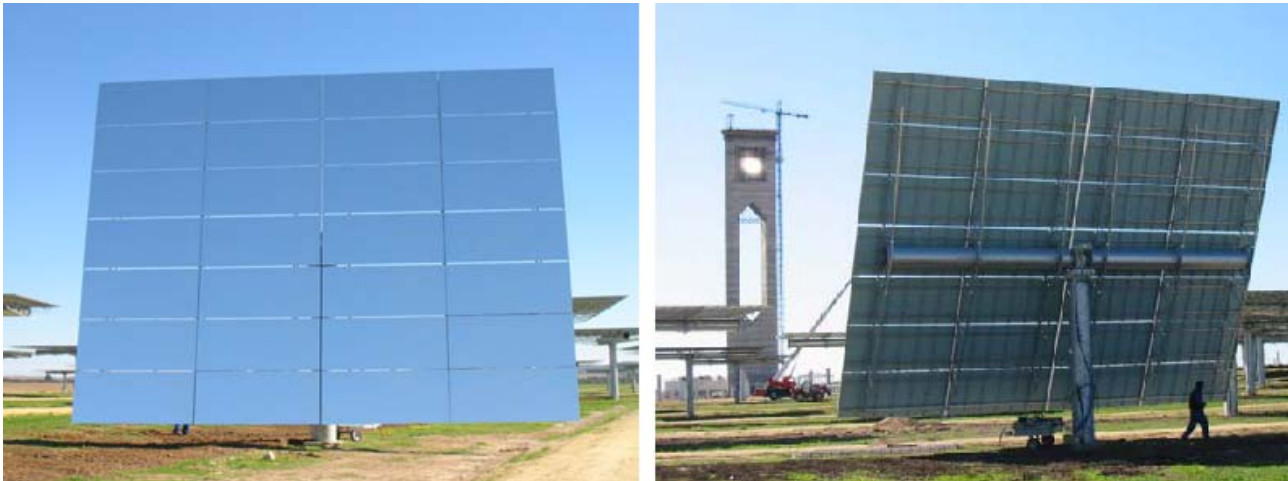
Figure 21: Heliostat of the PS10 Central Receiver Power Plant [PS10 Report 2006]
