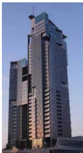
037 Ansicht Sea Towers [ © http://www.de.webtourist.net/poland/gdynia/sea-towers.php ]
