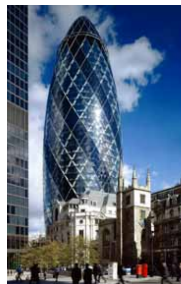
009 30 St Mary Axe (ehem. Swiss Re-Tower), London (Foster+Partners, 2003) [Gräwe 2006, 71.]
