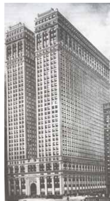
015 Equitable Building 1915 [Campi 2000, 14.]
