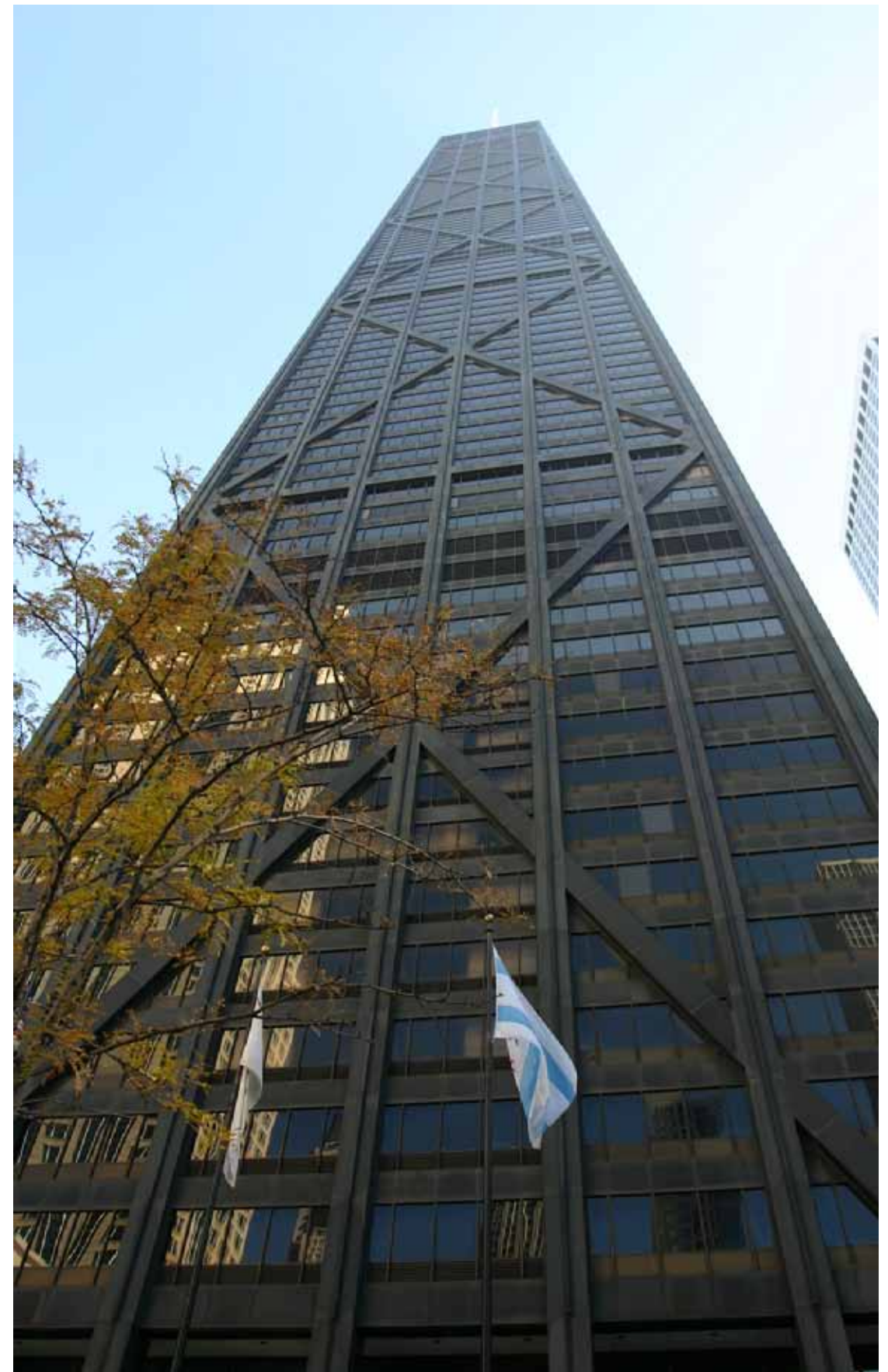
089 Ansicht des braced frame tube- Systems [ © Kuess 2010 ]
