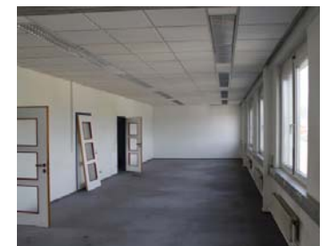
Fig. 27: Office and conference hall
