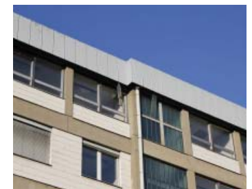
Fig. 17: Edge on the building
