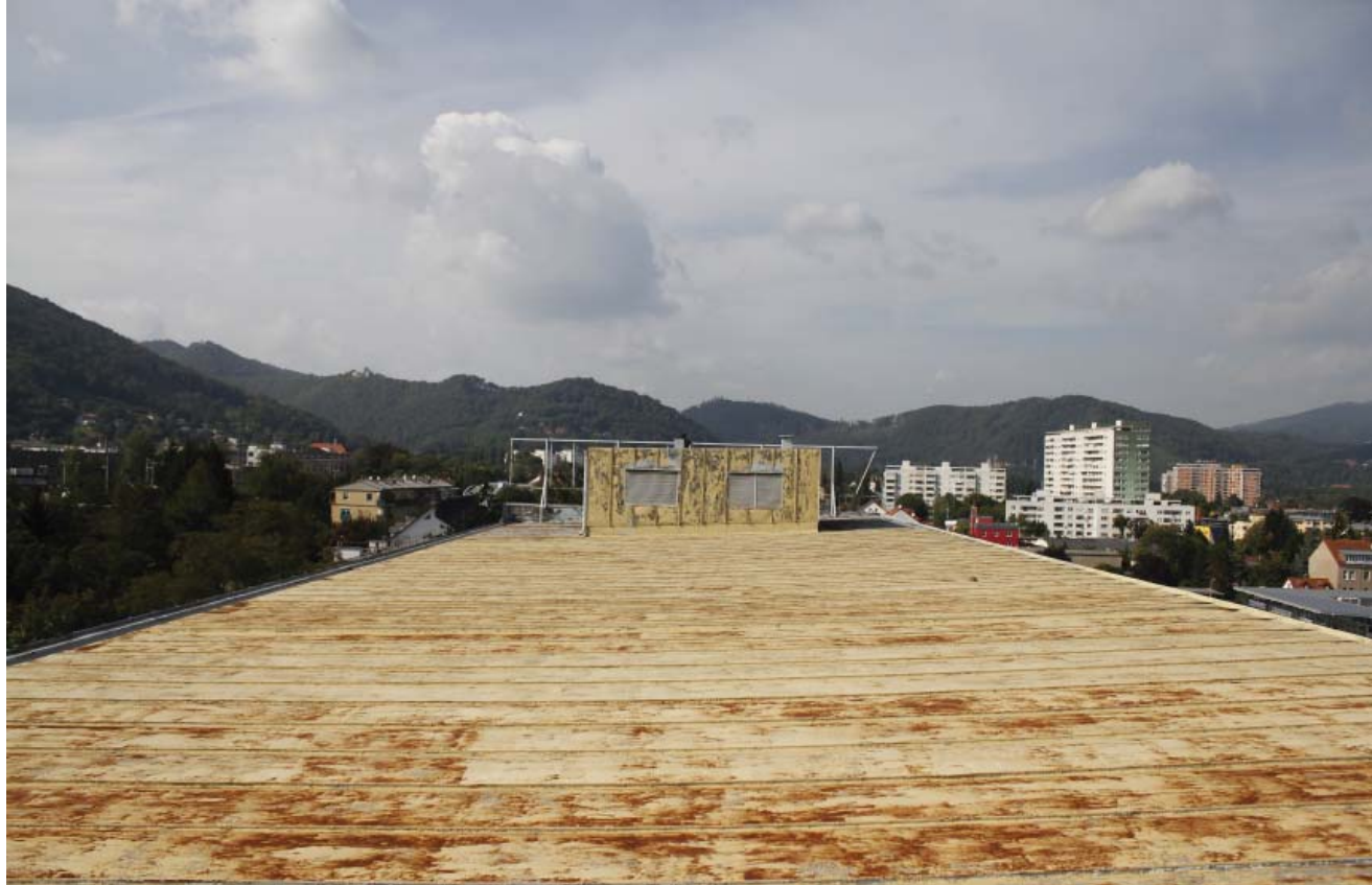
Fig. 54: View to the north on the roof of the building
