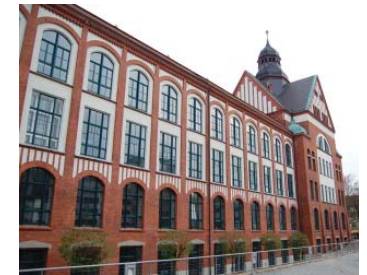
Fig. 76: Brickwork - stucco facade
