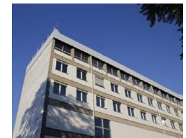
Fig. 41: Two sides of the building
