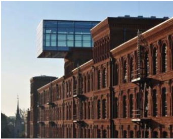
Fig. 83: Newly added glass roof
