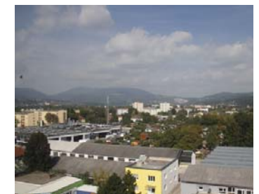
Fig. 112: View - seventh floor This image was taken on the last floor of the high-rise and illustrates the fabulous overlook over the district, which is very suitable for prospective apartments. The former factory had all its major office and conference rooms in the last floors because of this reason.
