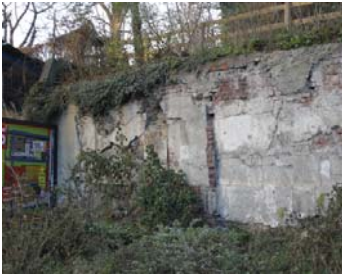
Fig. 113: Concrete retaining wall
