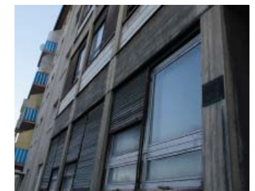
Fig. 46: Timbered window shutter
