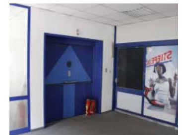
Fig. 21: Freight elevator first floor
