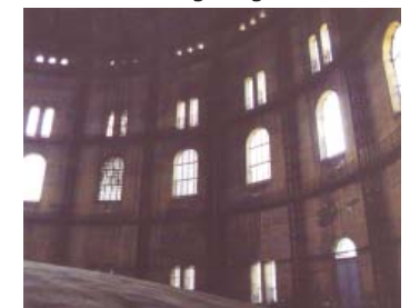
Fig. 60: Interior view on the wall
