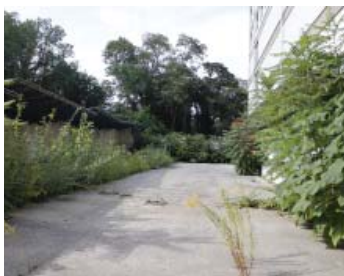
Fig. 9: Parking lot - backyard
