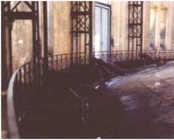
Fig. 61: Interior view - steel pillars
