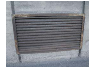
Fig. 32: Light wells - basement
