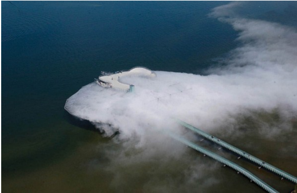
Abb. 33: Diller & Scofidio, Blur Building, Yverdon-Les-Bains, Luftbild
