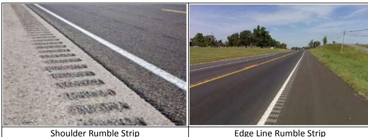
Abbildung 9: Shoulder Rumble Strip [14], Edge Line Rumble Strip [8]
