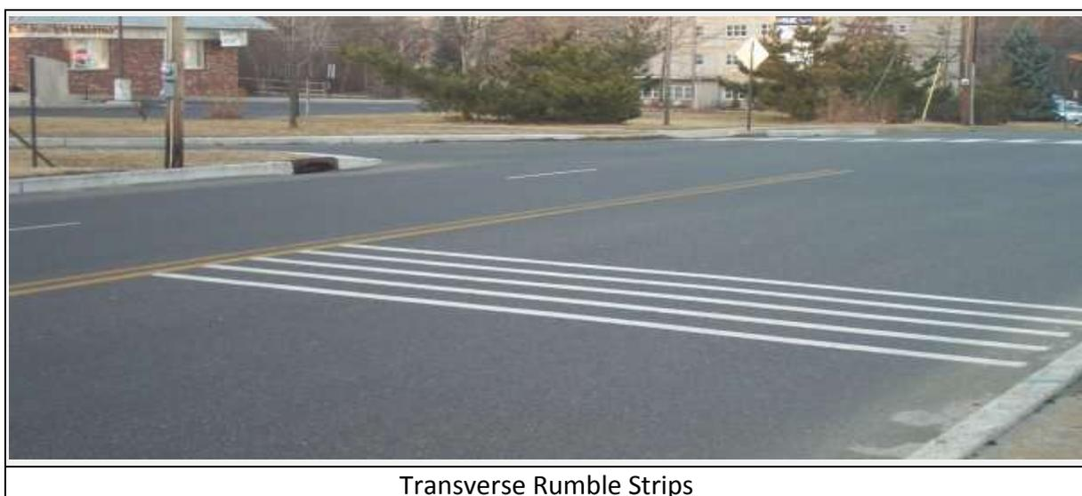
Abbildung 11: Transverse Rumble Strips [17]
