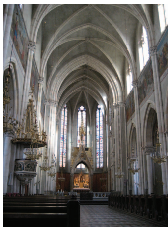
Figure 1.6: The nave of a baroque church is geometrically very complex. Acquiring a set of images that is sufficient for a complete reconstruction is a very challenging task.
