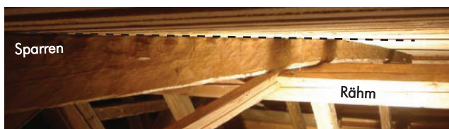
Fig. 4A.27 Trapezoidal portal frame in the hip area (see HÜBNER (2000)).
