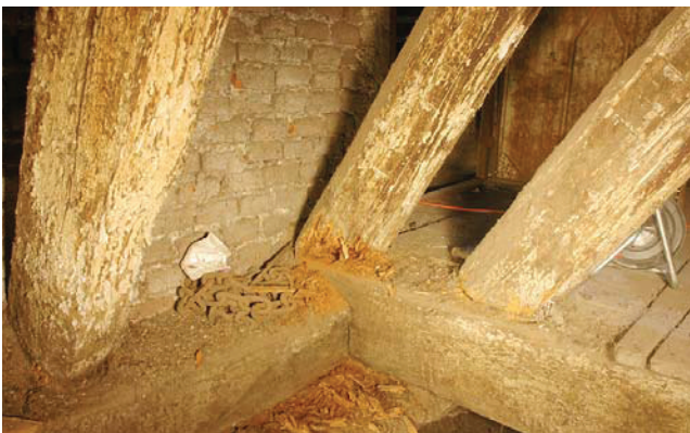
Fig. A.47 Top and bottom Left, top Right: damaged rafter base before and after working with the hammer tip, bottom Right: the wall plate is destroyed due to fungus inside (see penetration of the bar hammer).
