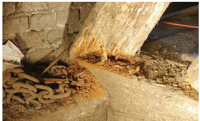
Fig. A.47 Top and bottom Left, top Right: damaged rafter base before and after working with the hammer tip, bottom Right: the wall plate is destroyed due to fungus inside (see penetration of the bar hammer).
