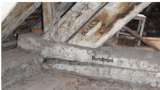
Bild 3.15 Querzugversagen des Bundtrams. Fig. 3.15 Failure of tie-beam due to stresses perpendicular to grain.
