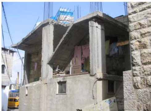
A: The steel bars that facilitate the planned future extension
