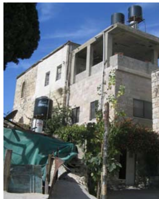
B: The newly added apartments on top of the old structure
