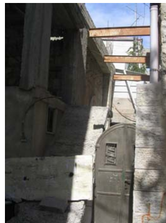
B: A new fixed metal door in the house's entrance
