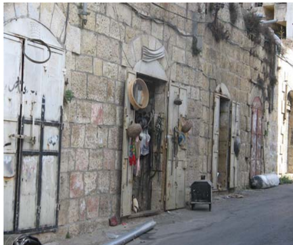
Figure 3.14: Commercial stores in a linear style, Al-Kundargiah Street (Author based on Al-Juabeh and Bsharah, 2002 )
