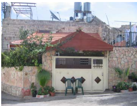
A: A new fixed metal gate
