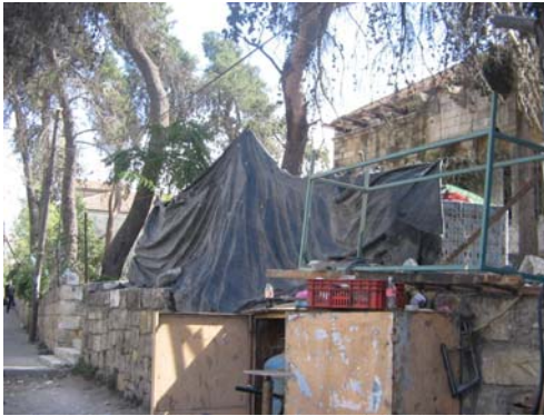
A: A fixed textile screen from the street side to provide privacy.
