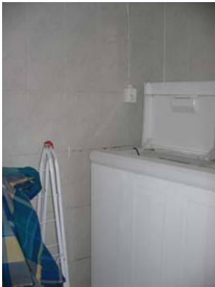
C: A newly added laundry room
