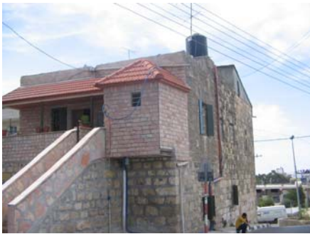
C: An added veranda and laundry room
