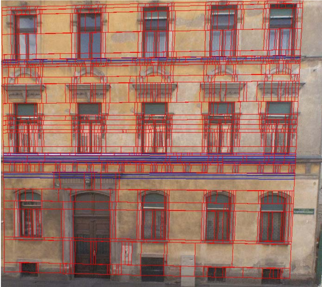
Figure 7.5: An example of façade division into set of blocks. Blocks are marked by red lines borders and each represents a uniform patch of the façade. Blue separator lines are detected from horizontal gradient image and indicate the presence of rims. Note that windows are divided into several blocks (window's planes, tops, frames, margins). In this façade, 1231 blocks have been detected, divided between 36 levels.
