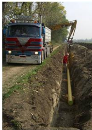
Figure 3.2: Burying of a natural gas pipeline, image by Ernst Schmutzer
