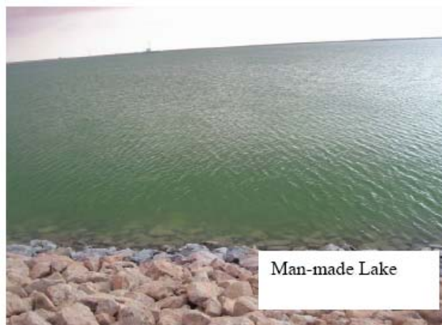
Figure 3.3: Man-Made Lake, Ommar Al Mochtar water reservoir, with storage capacity of 6 MCM and diameter of about 1 km (GMRA-Phase I).
