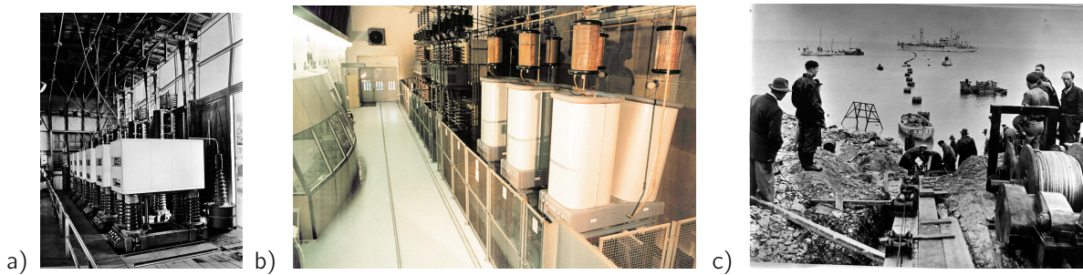
Figure 1.2: a) AC/DC Test installation in Berlin (1942) between suburbs of Charlottenburg and Moabit 2 b) Valve hall of Gotland 1 Line 3 c) Pulling the Gotland cable ashore 4
