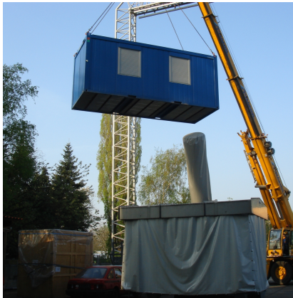
Figure 5.9: Delivery of Portakabin
