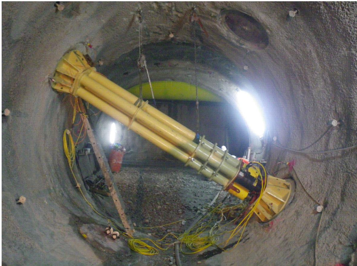
Figure 23: Assembled press unit.
