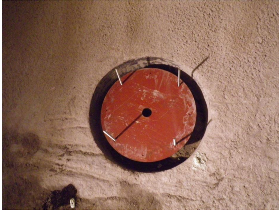
Figure 25: Mounted load plate on steel rods.
