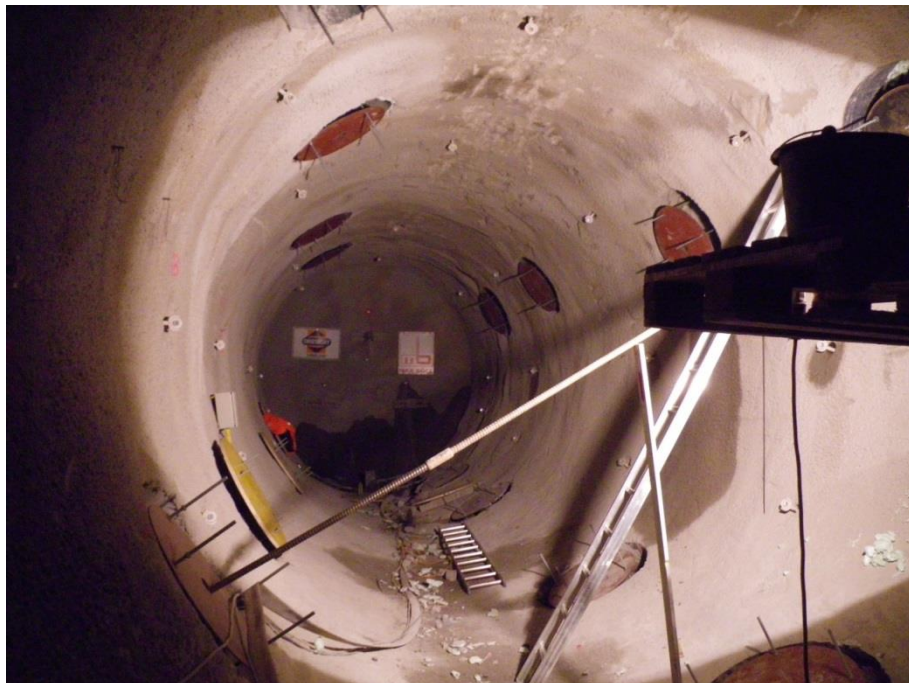
Figure 26: Load plates with mounted wooden plates as formwork (bottom left).
