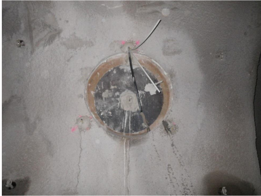
Figure 27: Grouted load plate and extensometers.
