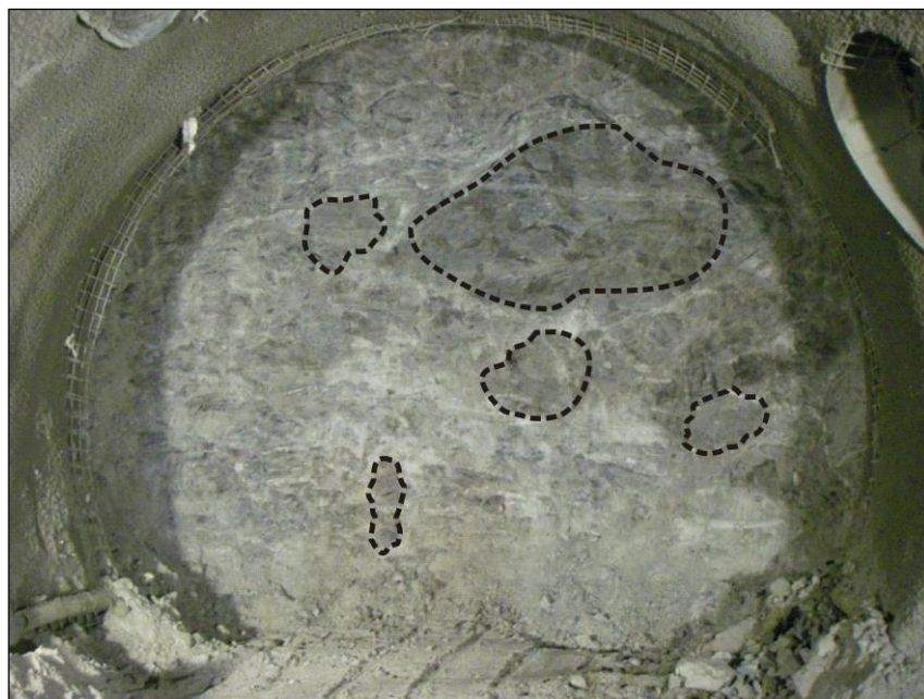
Figure 21: Geological conditions at chainage TM-VS 25.14 m; fractured schistose gneiss with competent rock blocks (marked with dashed lines) and cataclastic shear bands.
