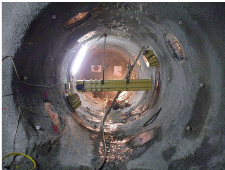
Figure 28: Set-up of the press unit by utilizing winch hoists.
