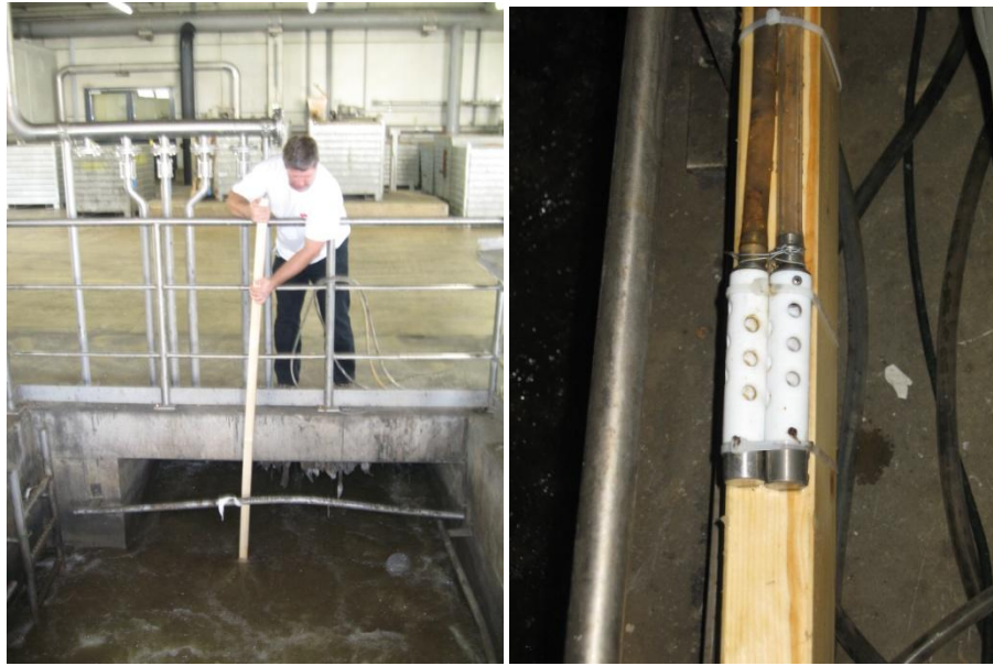
Figure 4.6: Assembly for collection of sample from Gravel Chamber
