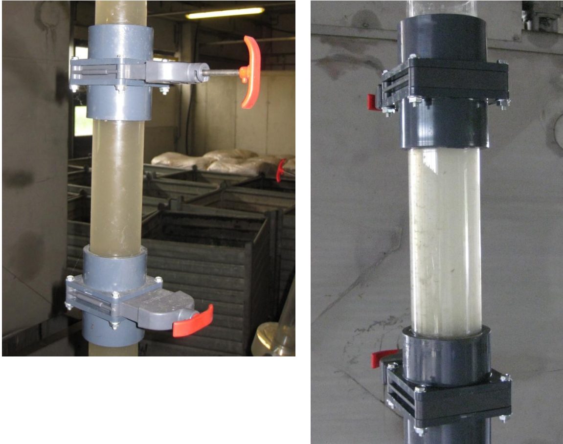
Figure 4.16: Valves of the settling column
