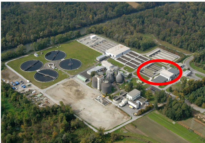
Figure 4.1: Target Area at Graz WWTP and sampling points
