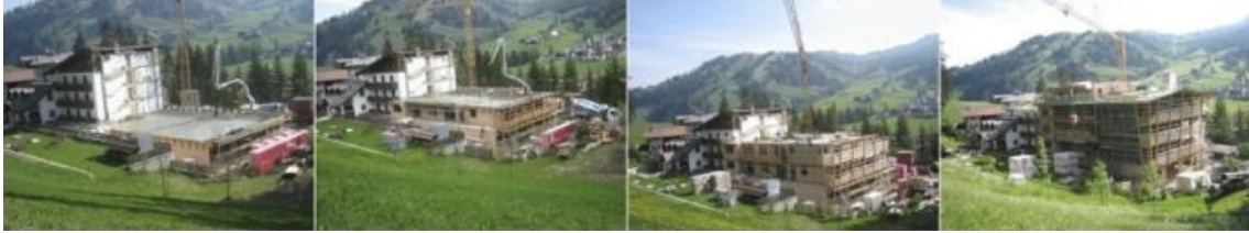
Figure 2.21: Construction site monitoring using camera images. The image sequence represents different steps of the construction progress.
