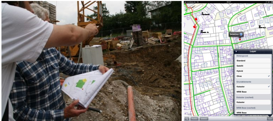
Figure 2.18: Traditional Methods for Information Query of Digital Assets. Left) Accessing information with a paper printout. Right) Accessing information with a mobile GIS interface.
