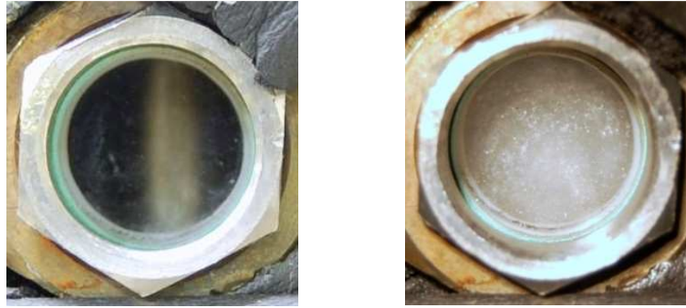
Figure 5-2: Photograph of a sight glass in the lower part of the evaporator without (left) and with NaOH crystals (right)
