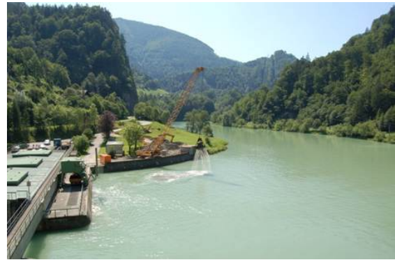
Figure 8.4: Dredging at the turbine inlets in July 2009
