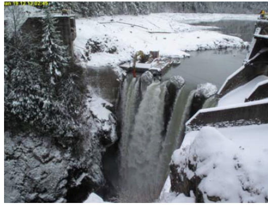
Figure 4.12: Glines Canyon Dam after deconstruction in January 2012 (USSD, 2012)
