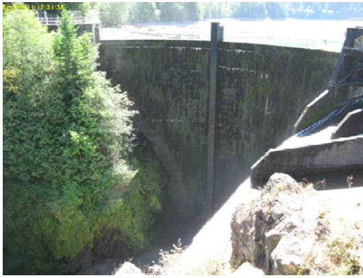
Figure 4.11: Glines Canyon Dam before deconstruction in September 2011 (USSD, 2012)
