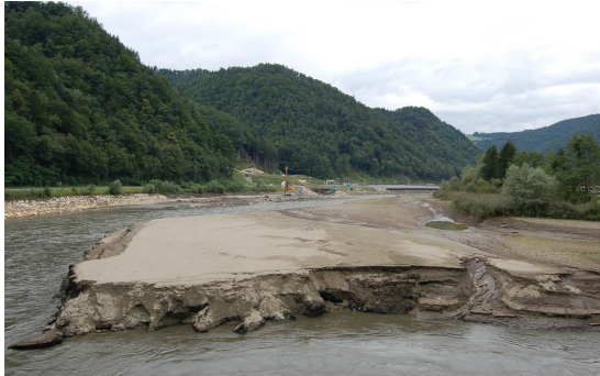
Figure 7.3: View from the weir of the Zlaten reservoir upstream with total lowering of the operation level due to rehabilitation works
