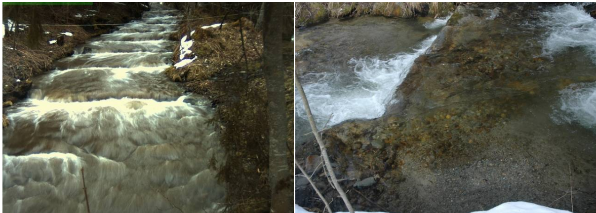
Figure 6.1 Melt Water Discharge on March, 25 th 2010, 18:27, CET (left), Sediment Sorting in Step-Pool Unit 4 of the Meandering Ramp (right)
