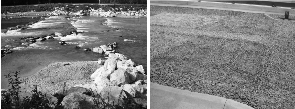
Figure 3.30 ramps with pool cluster: Saalach river, km 4.6 at low flow conditions (left), physical model of the Salzach river ramp, km 51.9 (right)
