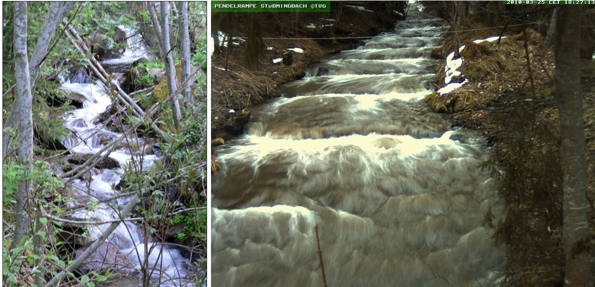
Figure 3.42 Natural model for the meandering ramp (left), first prototype meandering ramp, Stübmingbach (right)
