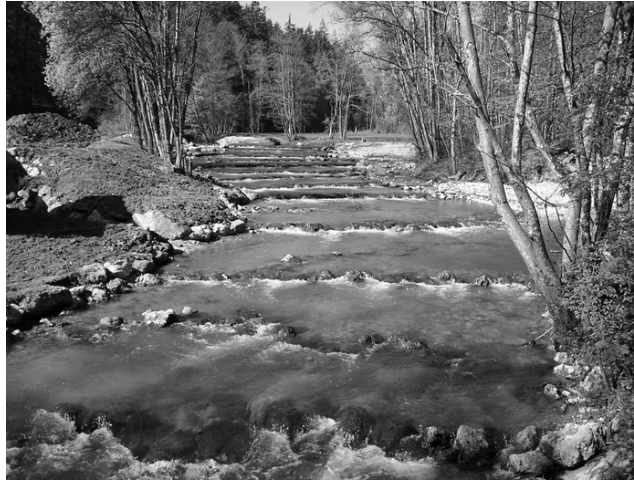
Figure 3.29 Example of a step-pool ramp near Teisendorf, Bavaria (© Wasserwirtschaftsamt Traunstein)
