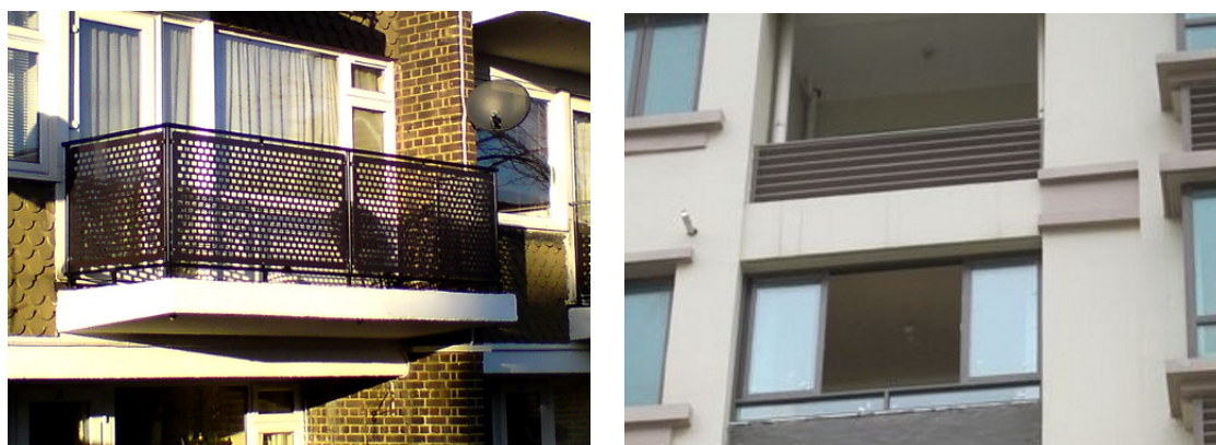
Figure 5.5: External open-sided balcony and internal balcony
