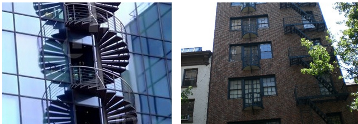
Figure 5.12: Outside fire stairs
