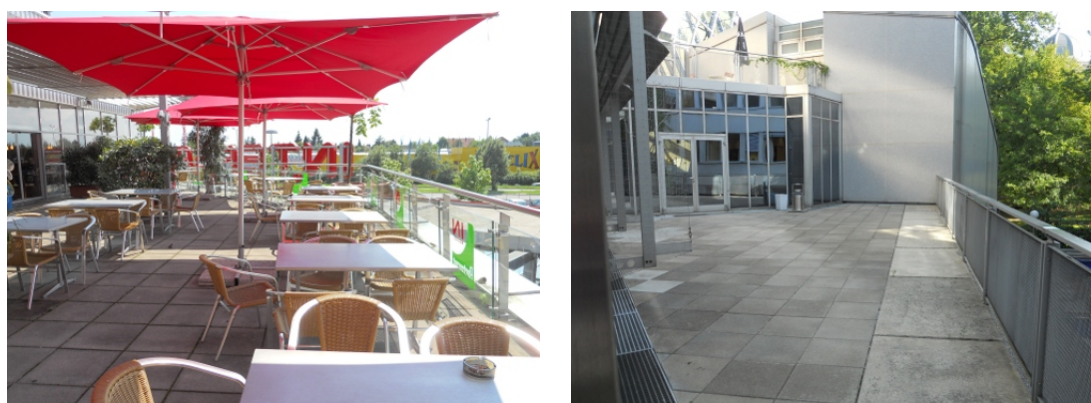
Figure 5.6: Uncovered roof terraces
