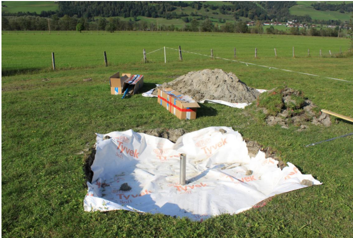
a) Preliminary excavation-covered with a membrane to prevent excessive evaporation.
