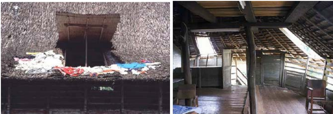
Figure 31. The skylight window on the roof to provide natural lighting and ventilation (Gruber et al. 2008)
