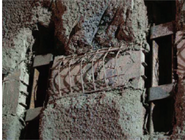
Figure 23. Installed hiDCon element (taken from Barla et al., 2007)
