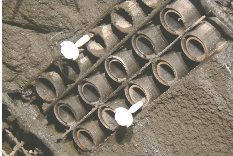
Figure 21. installed WABE elements (please note the inserted additional tubes)
