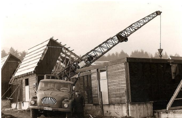
Figure 2-6: a.) On-site erection of single-panel wall elements in Varlovo housing estate in Maribor (1979), b.) Composition of TFCL 2 single-panel wall element.
