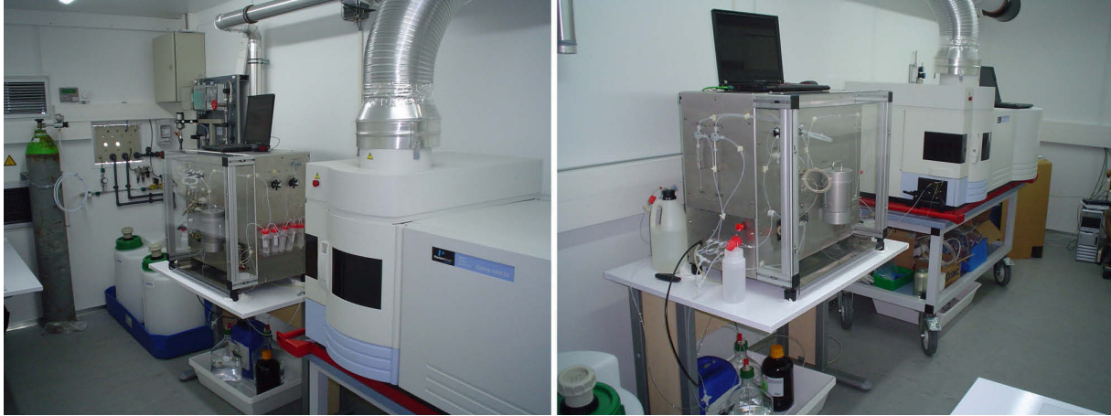
Fig. 6 - 15 Completely installed container ready for continuous operation
