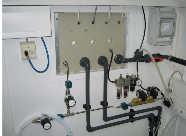
Fig. 6 - 2 Grey PVC tubing for sample supply (bypass) and waste line with connection board
