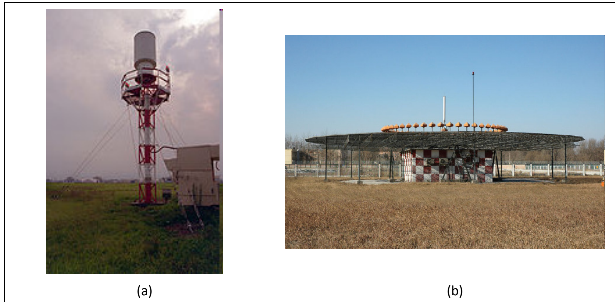
Figure 4-9: (a) TACAN station. (b) VOR/DME station (VOR antenna on the center pole). (source: US Air Force)
