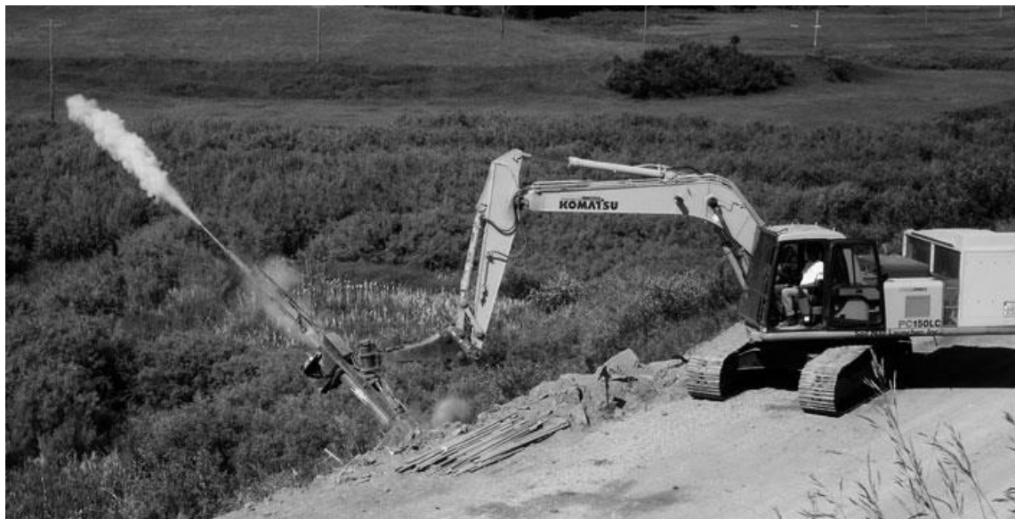
Abb. 21 Soil Nail Launcher™
