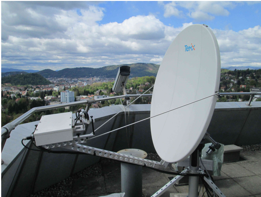
Figure 8: The Alphasat receiver setup at Hilmwarte tower.
