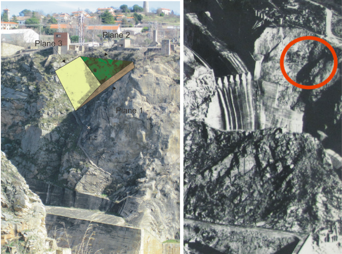
Figure 7.16 – Rock wedge moulds observed on the left wall
