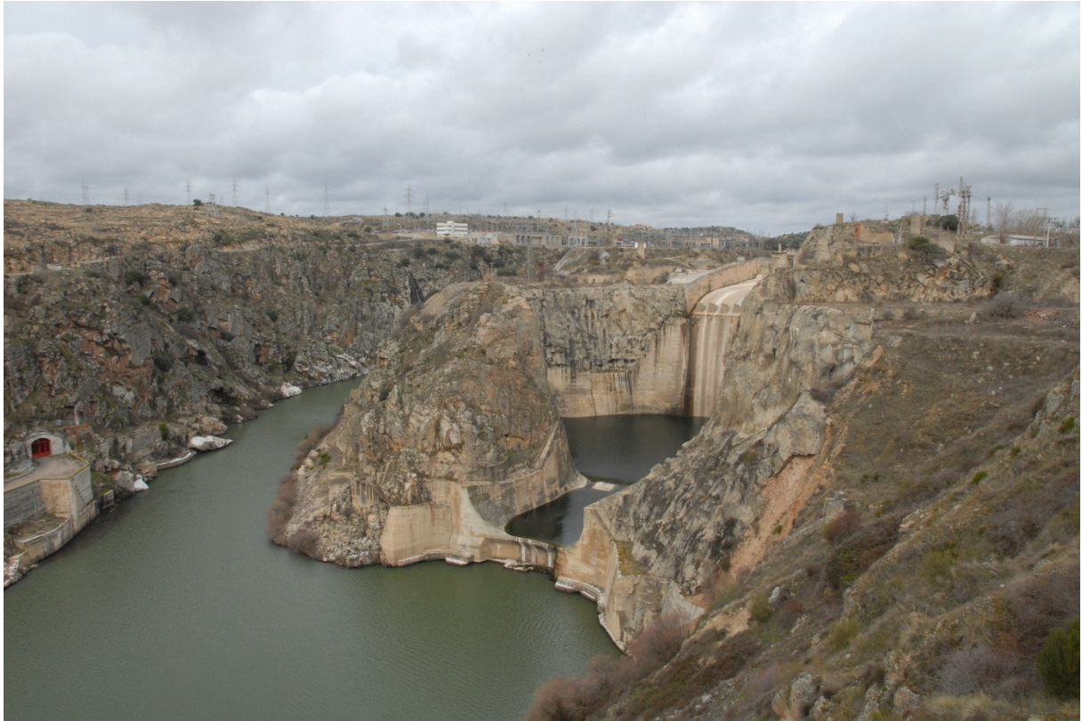
Figure 1.1 – The Ricobayo plunge pool
