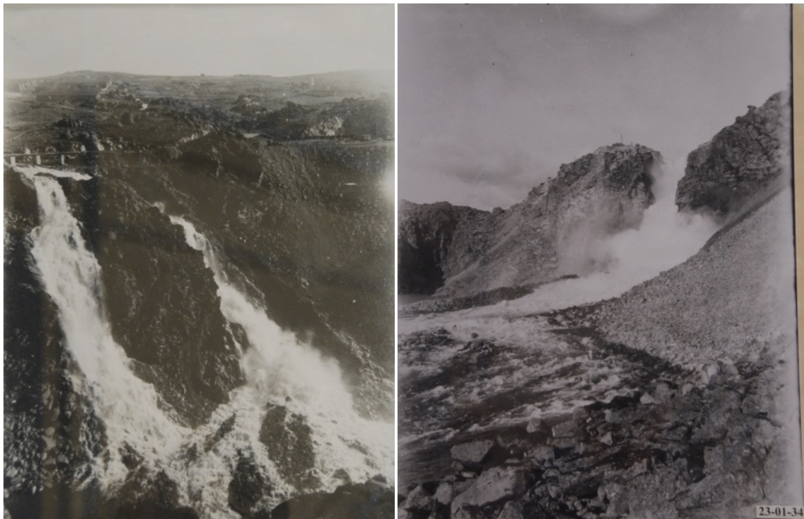
Figure 4.5 – Initial spillway operation (27/12/1933), and after first phase of the second erosion period (23/01/1934) – Iberdrola S. A.
