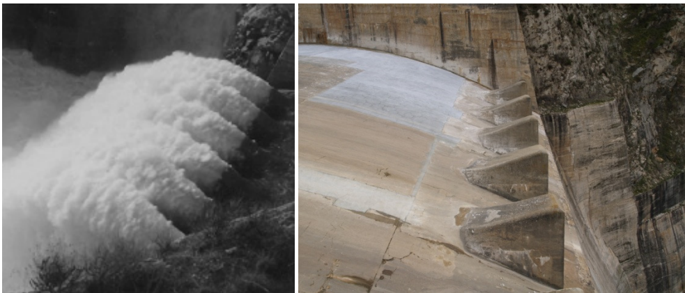
Figure 4.18 – Splitters at the spillway outlet (Annandale, 2005)
