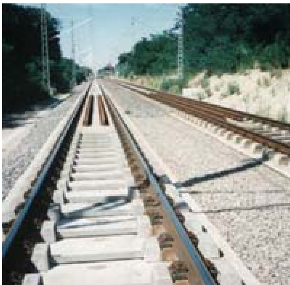
Picture 40: Track built in Züblin system
