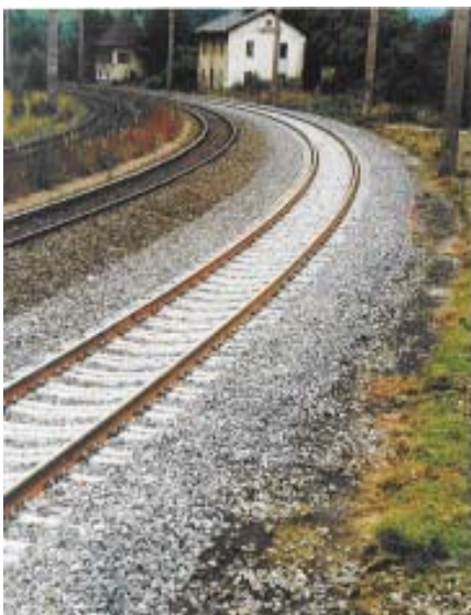
Picture 60: Frame sleepers in the curve and being installed 88
