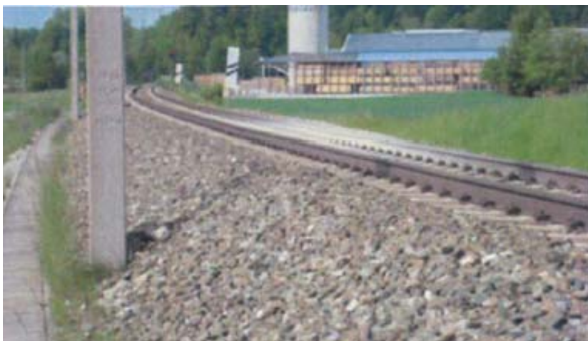
Picture 4: White spot due to ballast overloading
