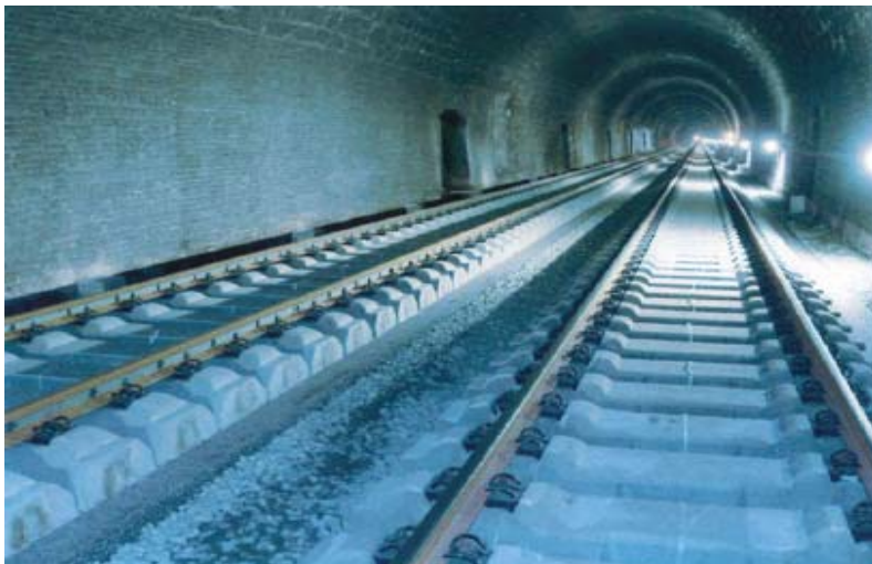
Picture 44: The finished GETRAC A3 ballastless track system 70
