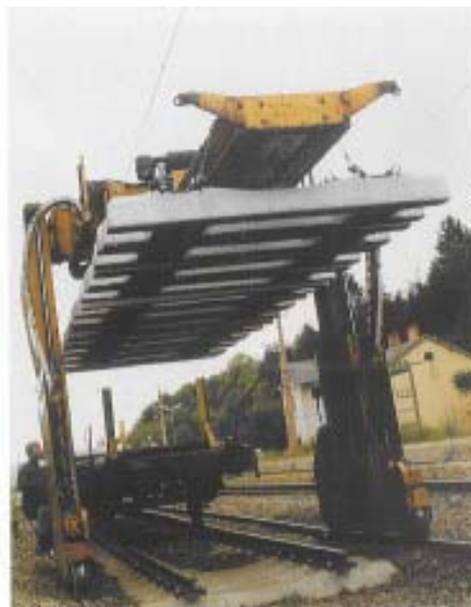
Picture 60: Frame sleepers in the curve and being installed 88
