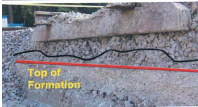
Picture 5: Cross section of the fines building up from the bottom
