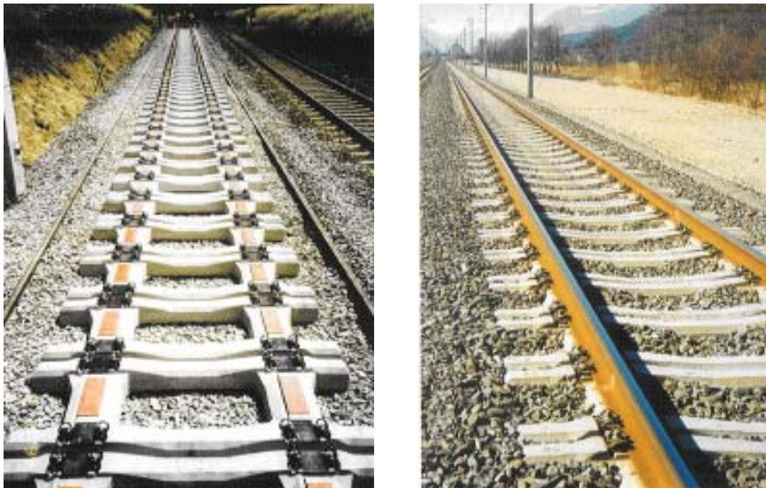
Picture 58: Frame sleeper on the ballast and on a straight line 83
