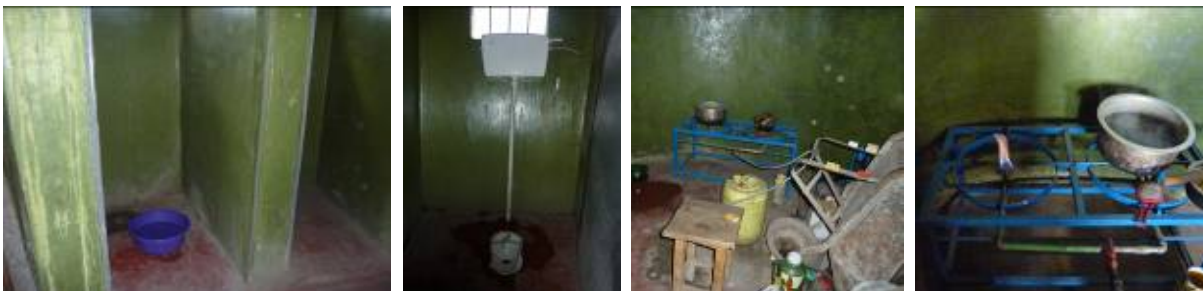
Figure 20 a - d. Interior of a bio-centre a) shower, b) flush toilet, c) and d) cooking device fueled by biogas (Source: Author)
