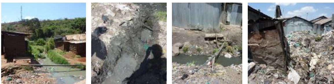
Figure 52 a - d. a) Water pipe and polluted river, b) and c) water pipes in sewerage, d) solid wastes on unoccupied land (Source: Author)
