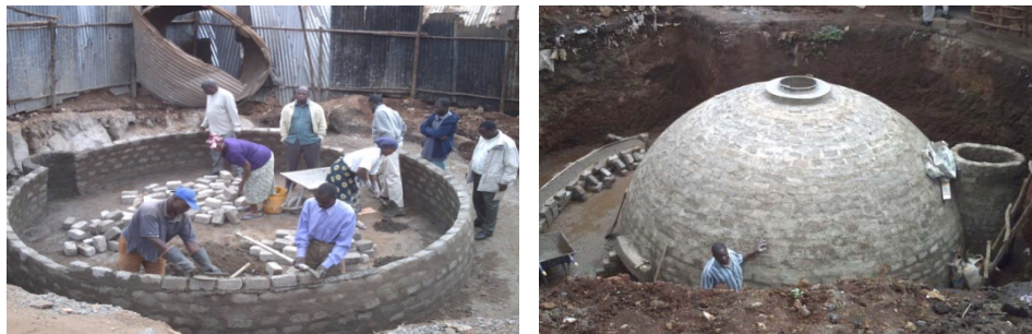
Figure 21 a - b. Working process in the construction of a bio-centre (Source: The Buckminster Fuller Challenge)
