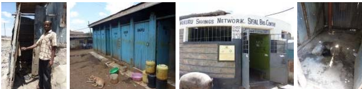
Figure 46 a - d. a) Plot-shared single pit toilet, b) community-shared single pit toilet with shower, c) bio-centre, d) inside a plot-shared single pit toilet (Source: Author)
