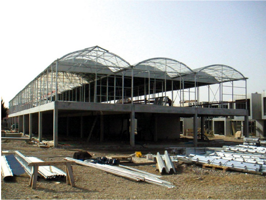
Abb. 29: Bauphase in Mulhouse
