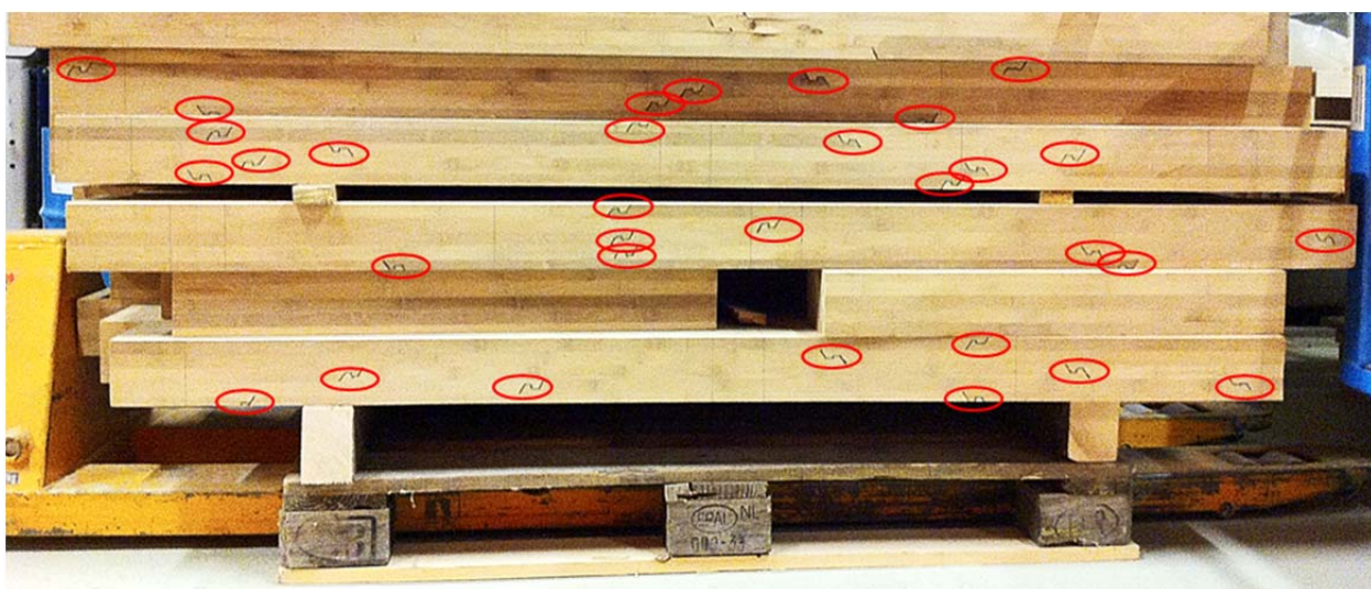
Figure 18: Beams with joints highlighted
