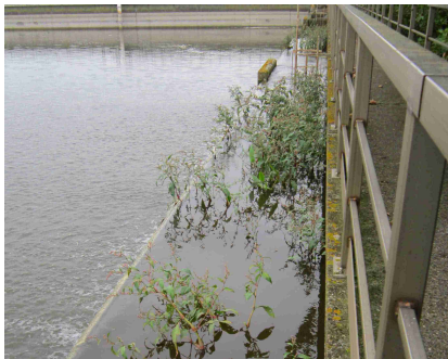
Figure 3.4: Photograph (left) and schematic illustration (right) of inlet structure: the raw water (A) is pumped into a vertical shaft (B), which is connected to a chamber of a horizontal channel, where the water enters the reservoir by an overflow weir (C). The plants visible on the photograph are not supposed to grow inside the horizontal channel.
