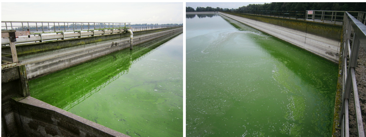
Figure 1.3: Dead zones and algal blooms inside the reservoir: dead zone at the outlet (left figure) and dead zone at a corner (right figure).
