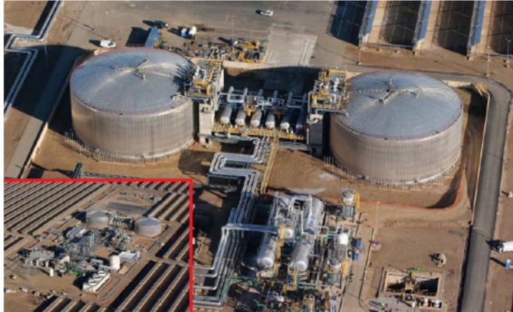
Figure 4-1: Andasol twin (cold and hot) molten solar salt storage tanks [78]
