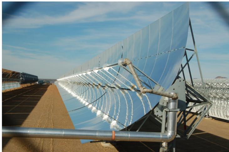
Figure 2-2: Parabolic trough receiver unit at Andasol-1, Spain [77]
