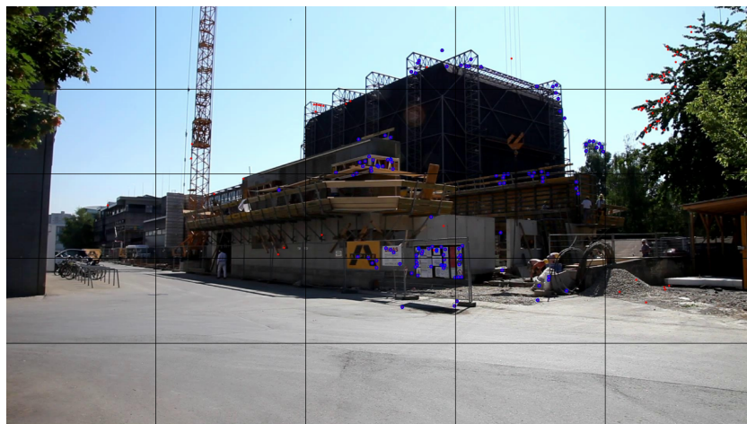
Figure 3.13: Illustration of the bucketing principle for an exemplar grid size of 5 \times 5 . First, n grid elements, also termed buckets, are selected randomly. Next, one element from each previously selected bucket is drawn randomly. With such a technique the probability of degenerated cases decreases.
