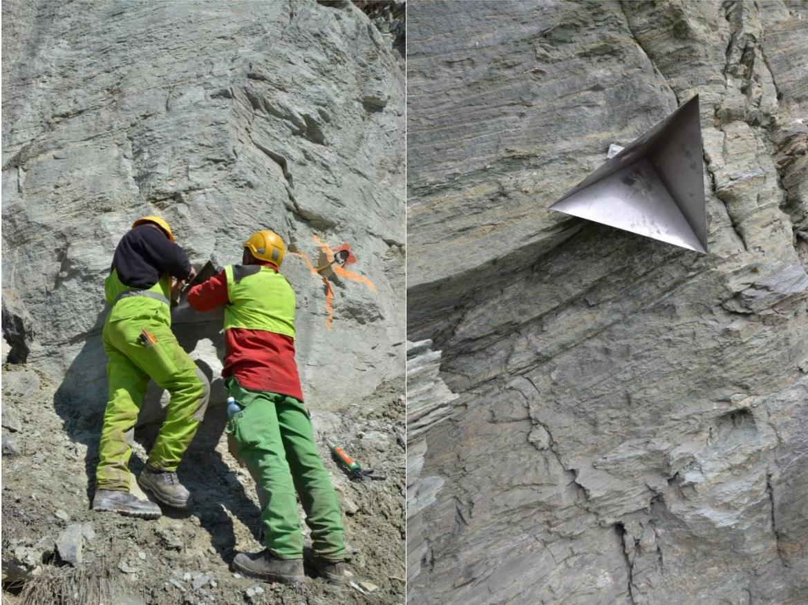
Figure 48, Installation of a corner reflector close to a fixed reflecting prism; Mounted corner reflector No. 8
