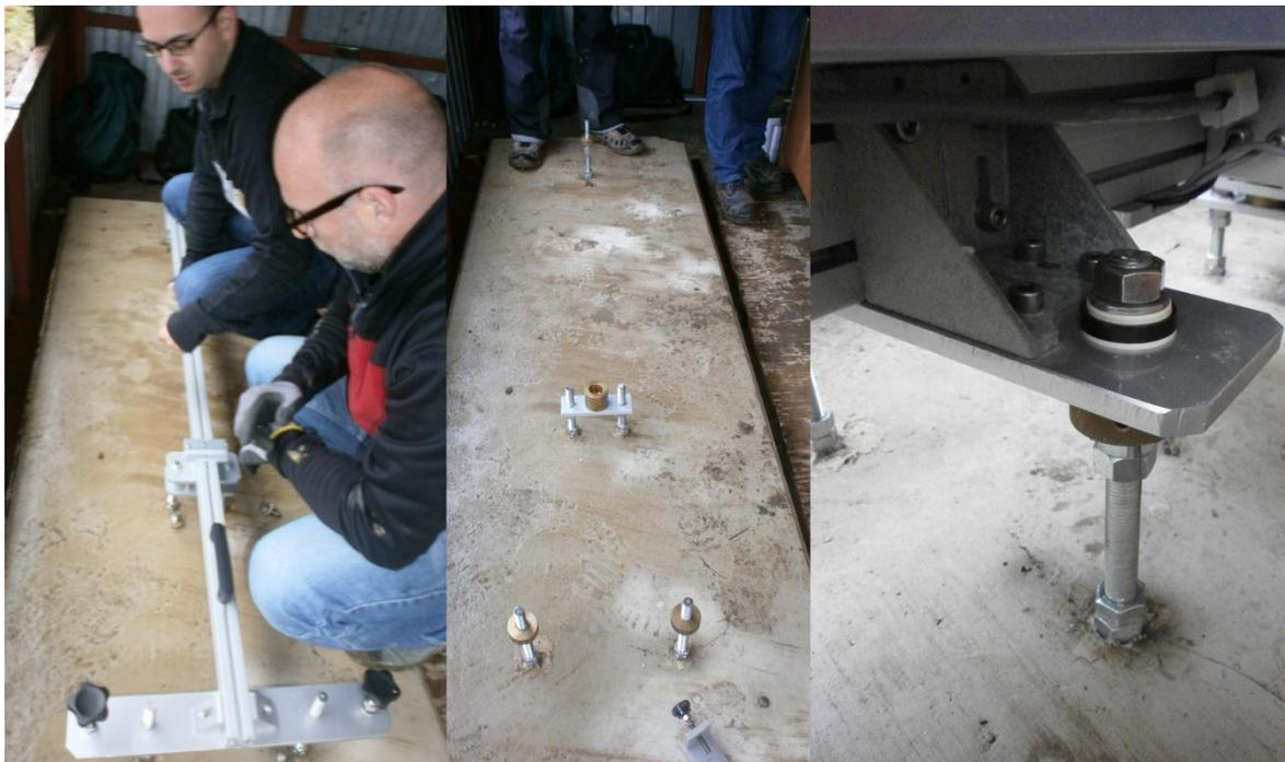
Figure 33, Using the positioning template for drilling the holes; resin injected holes with fixed threaded studs and base washers; detail of the installed rail.
