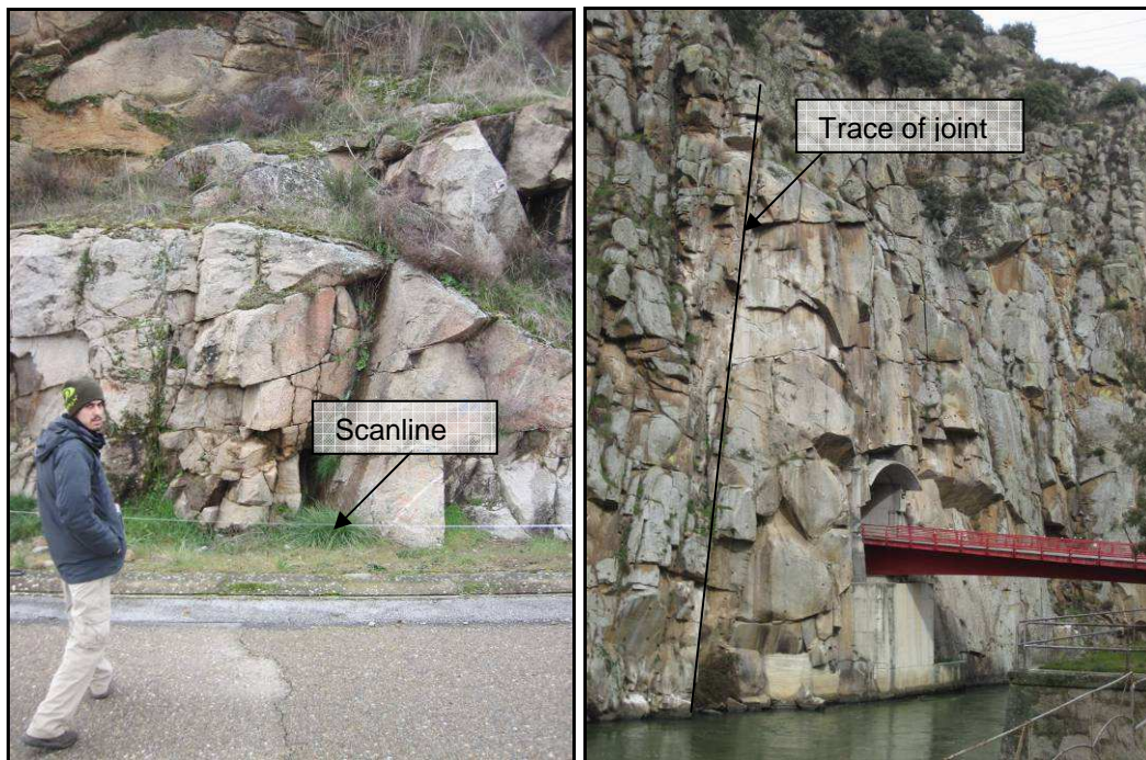
Fig.6 23: Outcrop situation at Ricobayo. Scanline along road cut (left). Estimates of the true persistence are difficult in this case. Large area of exposed rock along the river Esla right downstream of the dam (right). Some joints may be traced for more than 10 to 20m.
