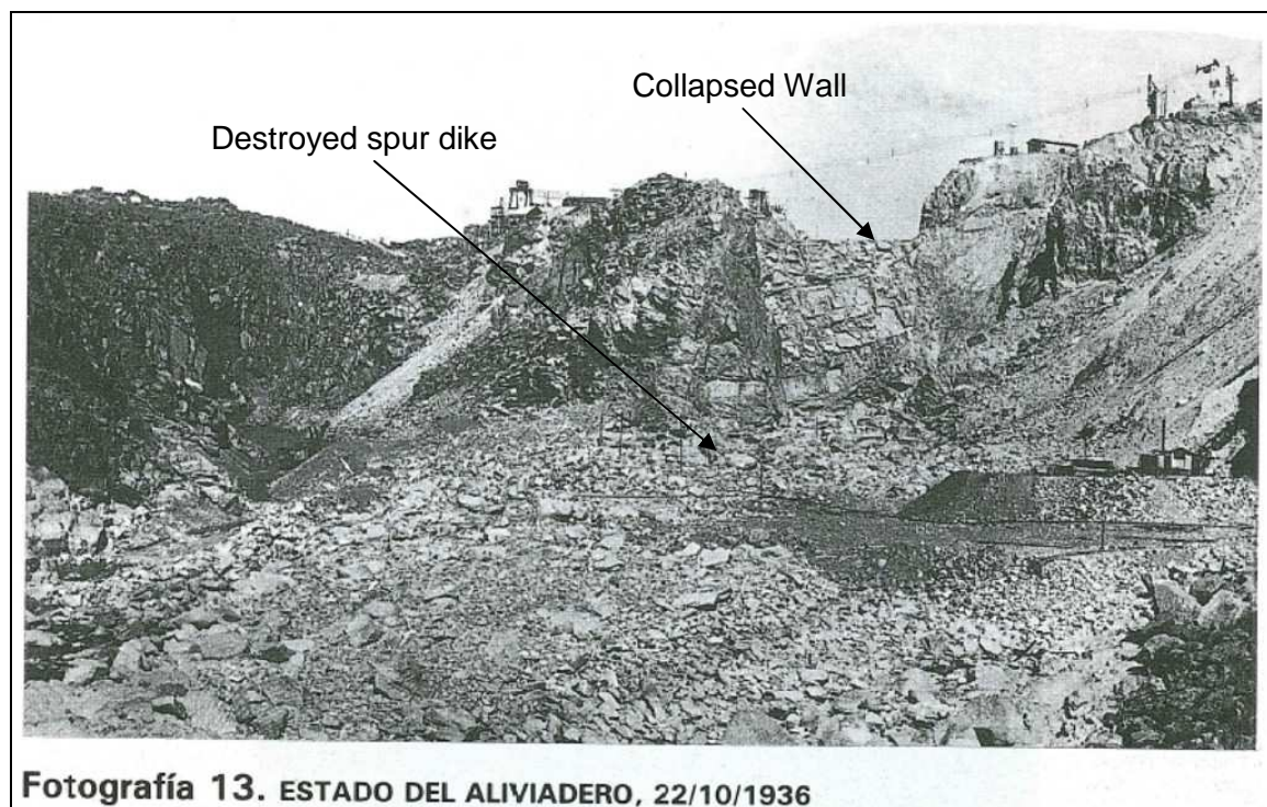
Fig.5 15: Collapse of the front wall of the spillway. View upstream where the front wall and the spur dike were situated at. Note the huge amounts of crushed rock in the riverbed (Guia tecnica, 1997).
