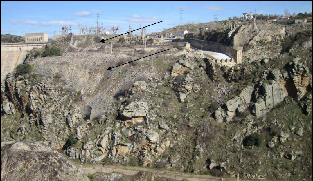
Fig.6 13: View to the area between the spillway and the river. The finer material dumped down on the left side of the picture forms fill deposits (arrows) for creating construction space. Location of the deposits is illustrated in Fig.6.12 above.
